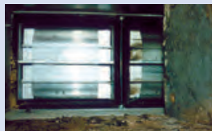
Photo 4C: Moldy air duct
