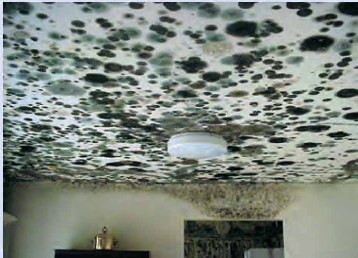
Photo 2: Extensive mold contamination of ceiling and walls
