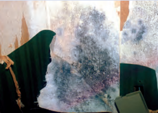
Photo 5: Mold growth behind wallpaper
