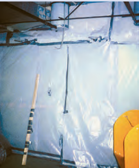
Photo 8: Full containment on large job
