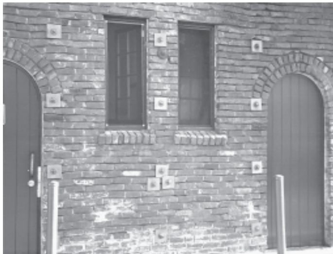
Figure 28 - Bolting of unreinforced masonry wall to steel frame on the inside.
